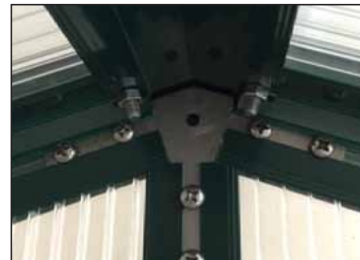
Interior greenhouse view of mid roof cap, where Z06 screw goes through WG01 mid hole into the end cap.
