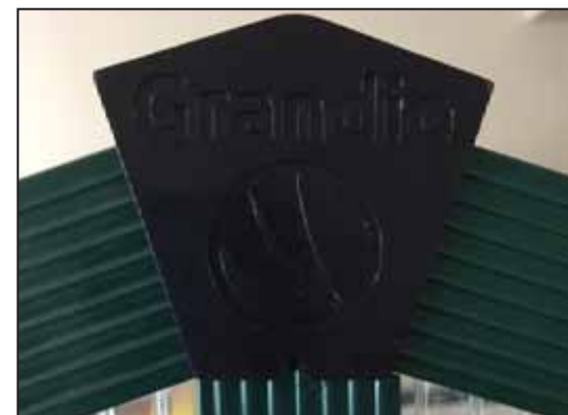
Exterior view of mid roof cap JG01.
