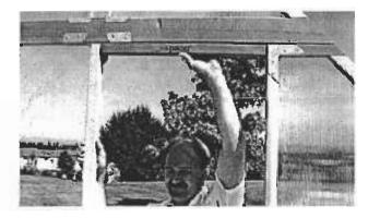
Attach the stud through the connectors using 3/4" screws.
