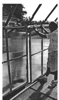
Swing the "halfway connected" second and third panels inward and press them together into alignment with the base.
