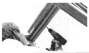
From the inside the GardenHouse, secure the unvented panels using 2-1/2" screws through the three **pre-drilled** holes in the ridge.
