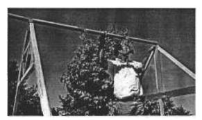
Rest the **ridge front** onto the front wall and center truss. With the ridge flush with the front wall, attach it through the connectors using 1-1/4" screws.
