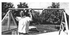
(If not already done at the factory, rest the ridge front and ridge back pieces on the side wall top plate with the connectors pointing down. With the ends of the ridge flush with the ends of the top plate, mark with a pencil on the inside of the top plate at the front of each
