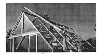
Repeat this procedure for the **center roof panel** and the **back roof panel**. The back panel will overhang the back wall 3/4".
