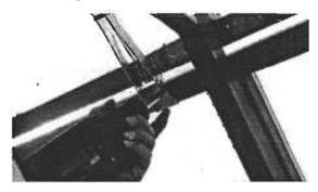
Position a vent operator near the center of a roof vent along side a truss with one bracket on the vent frame bottom and one on the adjacent roof panel blocking. Attach the two brackets using four 1-1/4" screws.
