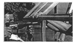
Drive 1-1/4" screws through connectors on the outside, lifting any sag from the top plate.
