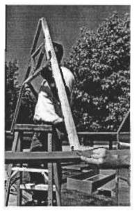
Slide the **ridge back** into the center truss connector and resting on the back wall. With the ridge flush with the back wall, attach through the connectors using 1-1/4" screws.
