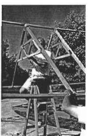
Seat the remaining four trusses fully into the connectors. Attach them to the ridge using 1-1/4" screws, and to the side wall top plates using 3/4" screws through the **untaped** holes.
