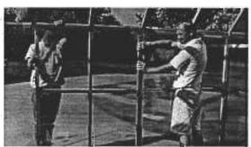
Position the second side wall panel at the edge of the first panel. Drive 2-1/2" screws halfway into two **pre-drilled** holes along this joint.
