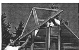
Drive 2-1/2" screws through pre-drilled holes at the roof line joint.
